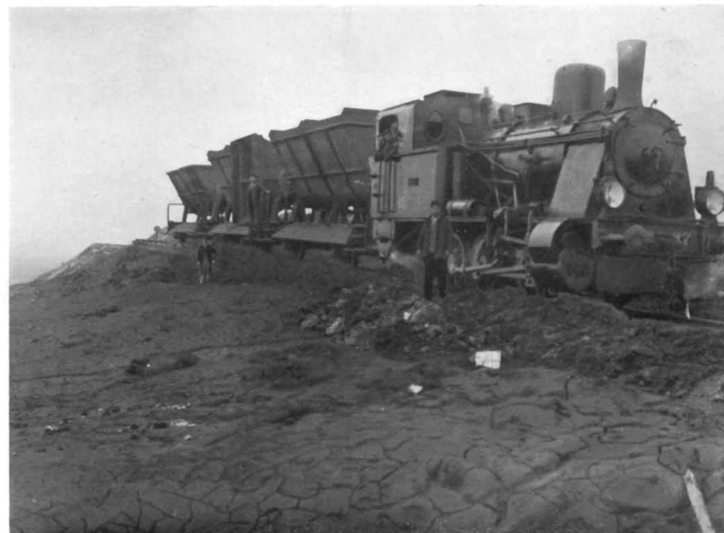
Fig. 3. Dumping of flocculated sludge. See cracks in dried material in foreground.
