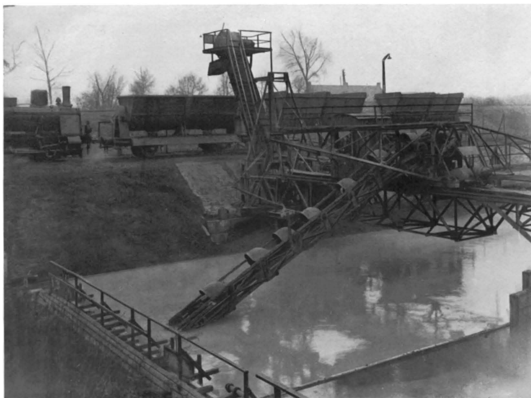
Fig. 2. Detail-view of bucket dredger, rubber-belt conveyor and elevator for charging dumping cars with sludge flocculated with lime.
